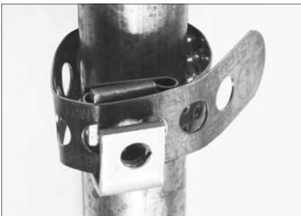
Step 11 - Wrap Strap Tight Around Pipe
