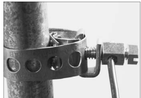
Step 13 - Insert Wire Into Hole & Install Bolt / Tighten Bolt against Wire using 10mm Wrench, Ensure all is Secure
